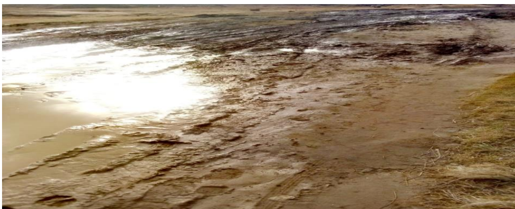
Image 4.8.2 (a) A dirt road in Motheo after some rain fall
