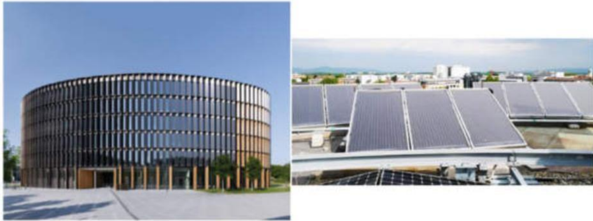
Figure 13: Façade integrated PVT system (left) and roof-integrated PVT system (right) [32]
