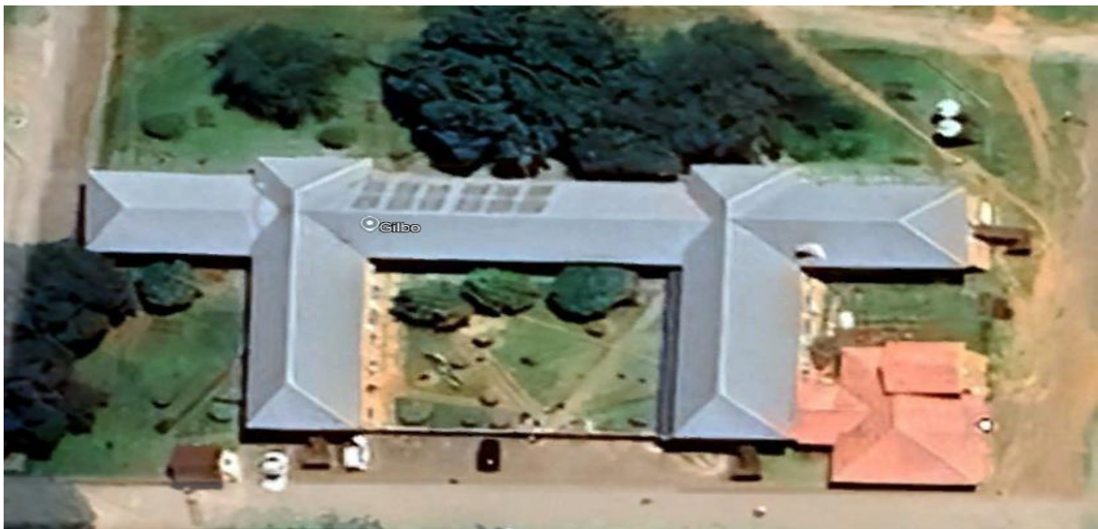
Figure 18: View of the NUL student residence known as Gilbo
