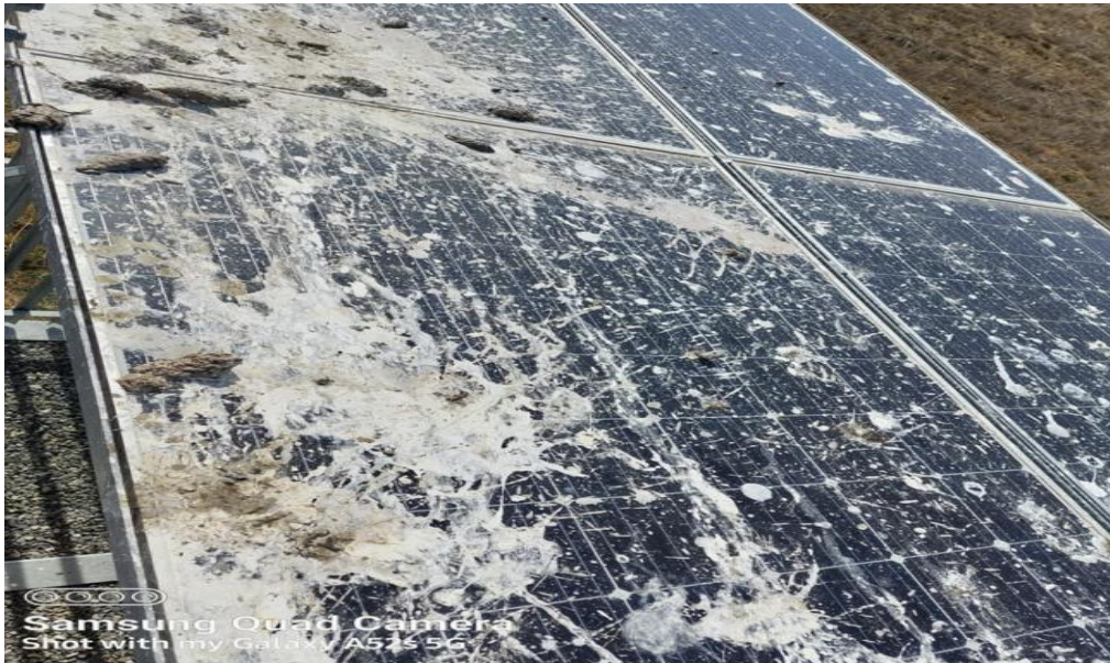
Figure 5: Solar PV plant at Vodacom Lesotho's tower located in Qopo, Mokhotlong
