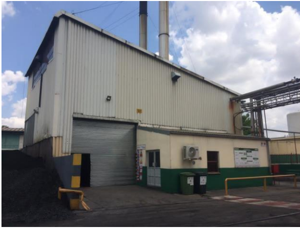
Figure 20: Boiler house at MMB with a heap of coal in front of it
