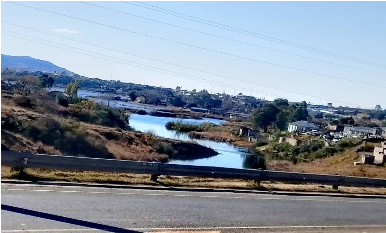
Plate 4.4. Maqalika Dam Upstream. Source: Author (2025)
