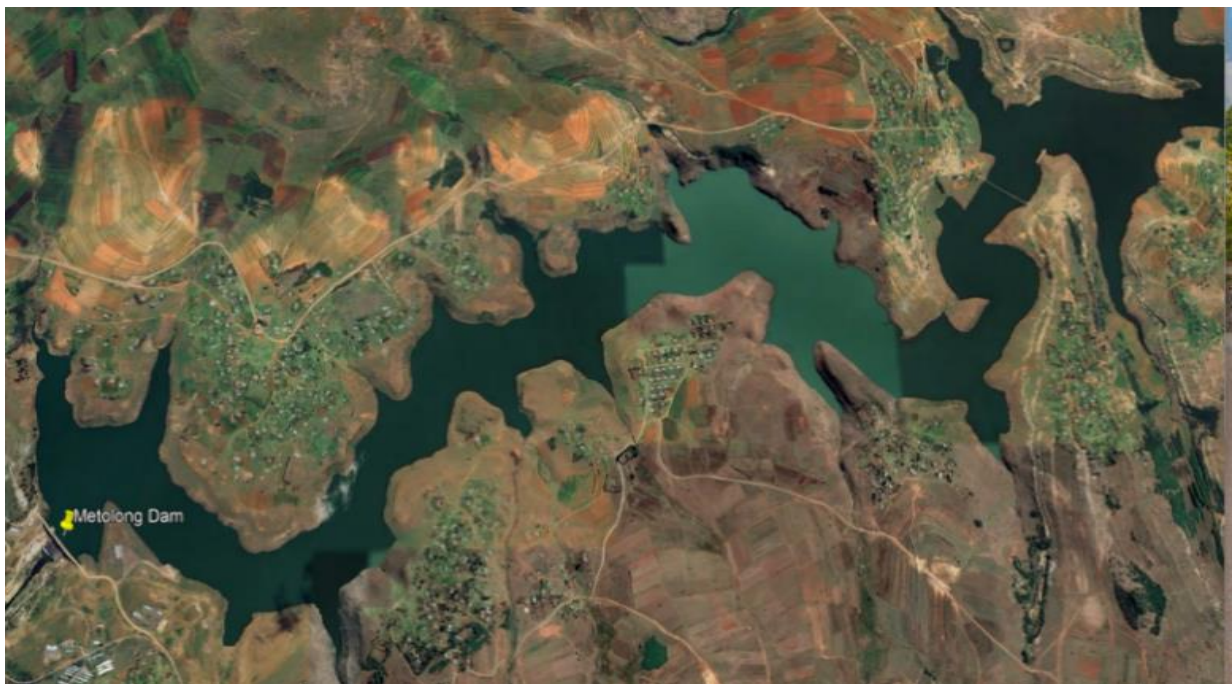
Figure 4: Image showing land uses around the reservoir (Google Earth Pro, 2024)
