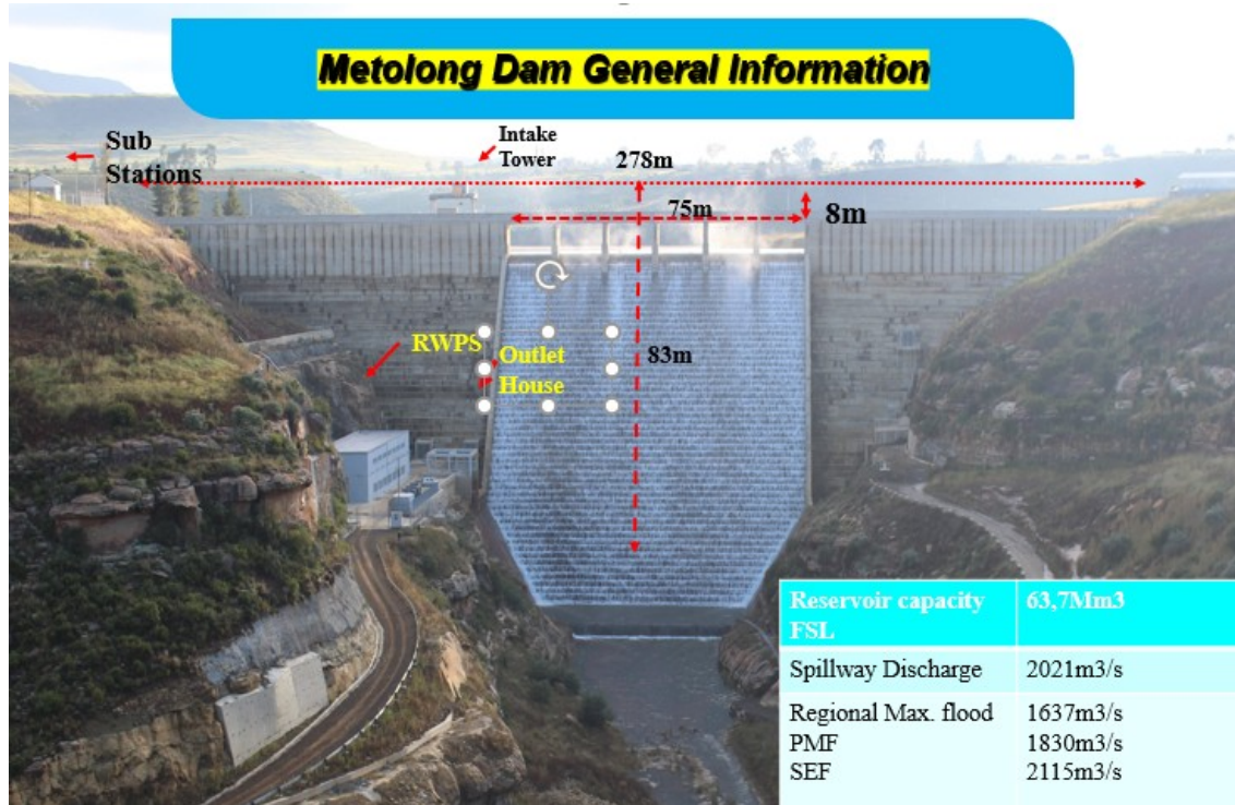
Figure 9 : Metolong Dam wall general information (Source – Metolong Dam Safety Department).
