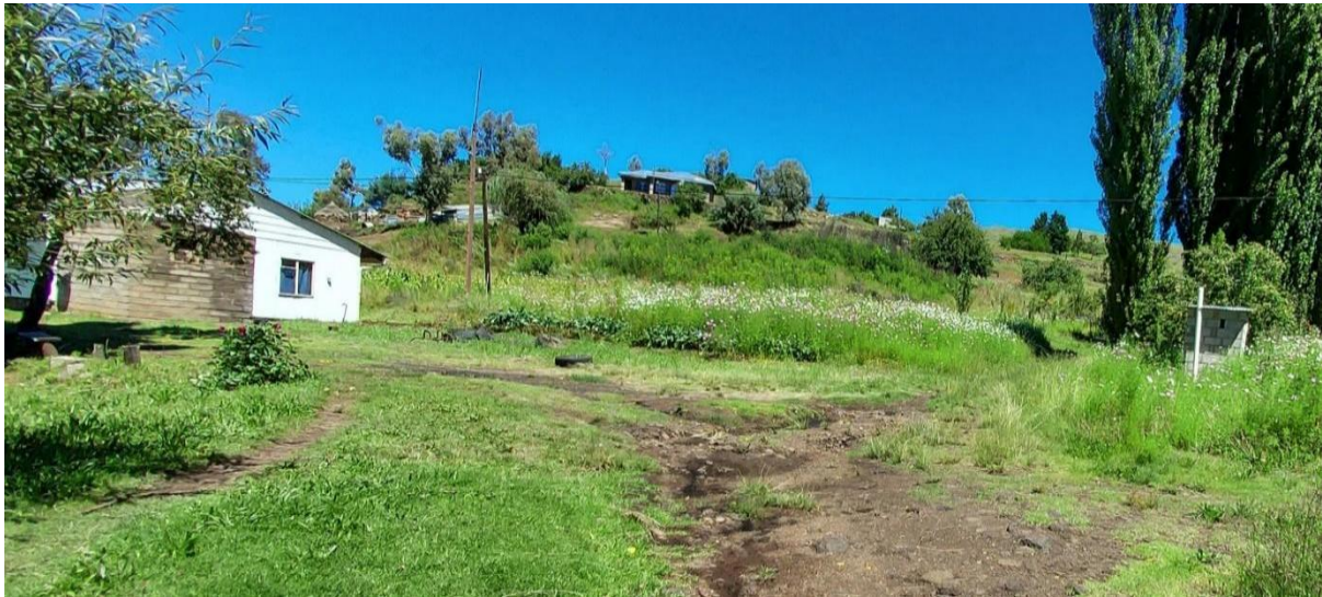
Figure 10: Refurbished office and a newly constructed toilet
