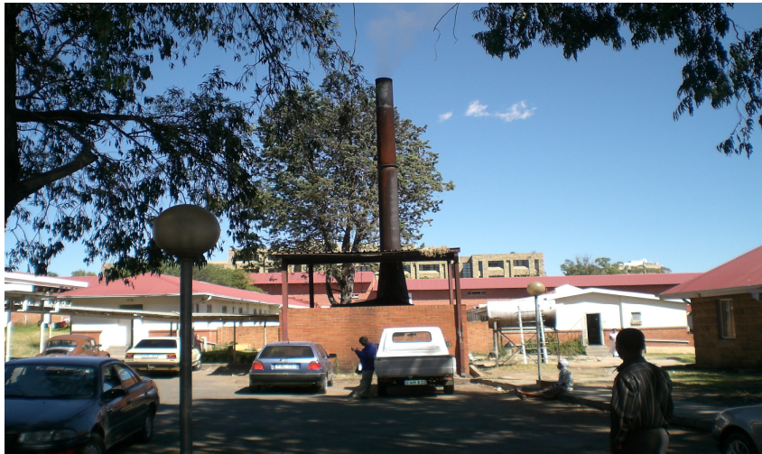
Plate 4: Queen II Hospital Incinerator
