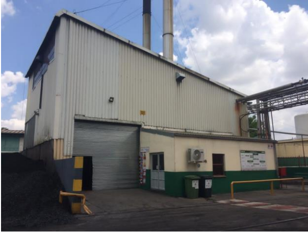
Figure 20: Boiler house at MMB with a heap of coal in front of it
